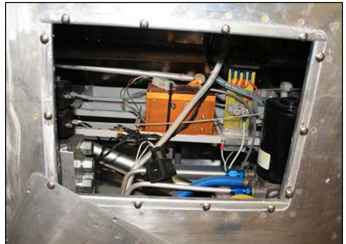
T-51 Utility Bay. Hydraulic manifold left, accumulator right , auto pilot rear.
