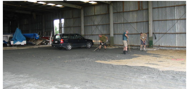
ARMAC preparing to concrete the floor of the packing shed.
